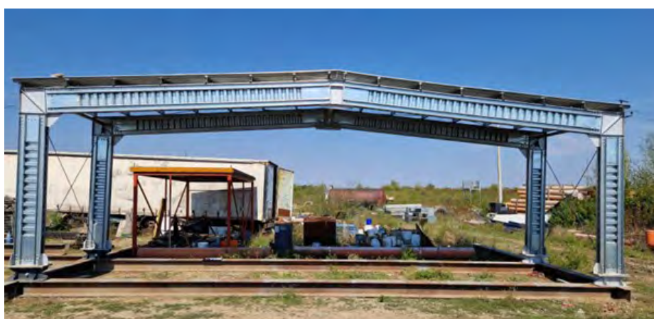
Single-storey industrial buildings made of cold-formed steel beams with corrugated webs
